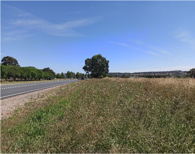
Picture 1 Existing street condition along Holbrook Road
